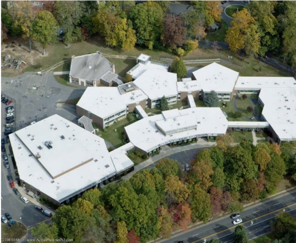
Low-slope roofing membrane installed using low-VOC adhesive and consisting of a modified bitumen cap sheet and base sheet.
