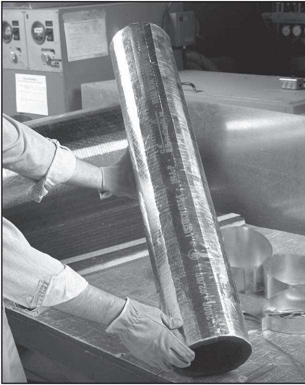
Figure 5-20. Completed insulation section with longitudinal seam taped
