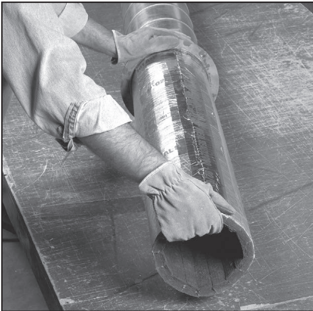
Figure 5-21. Slide insulation section into metal duct
