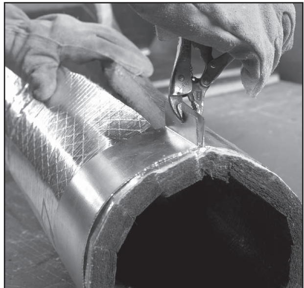
Figure 5-16. First draw-band in place with clamp
