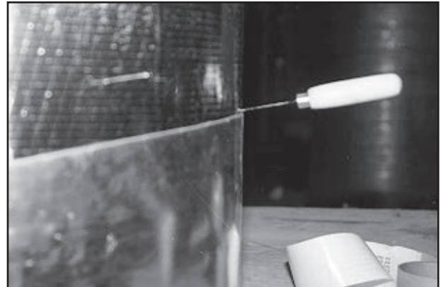
Figure 7-4. Cut liner with insulation knife
