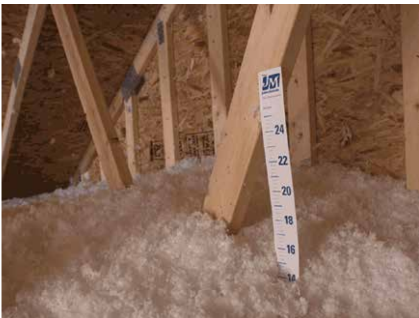
Installed blowing wool
