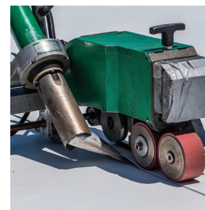
Heat Welding Seams
