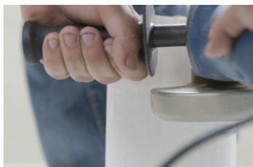
1. Abrade & Clean the substrate
