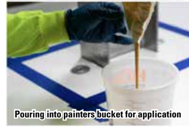
Thorough mixing of Component A & B
